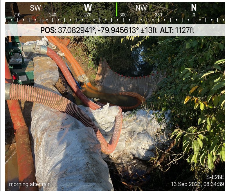
Photo Description: Next day additional pumps and dam reinforcements installed.
