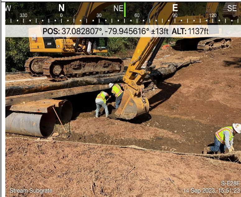
Photo Description: Restoration of stream substrate to channel.
