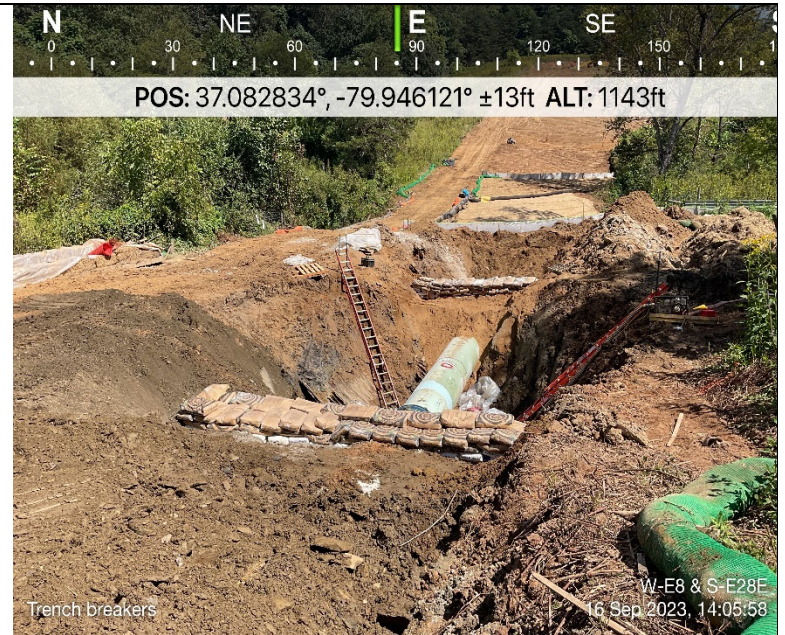
Photo Description: Trench breaker installations.
