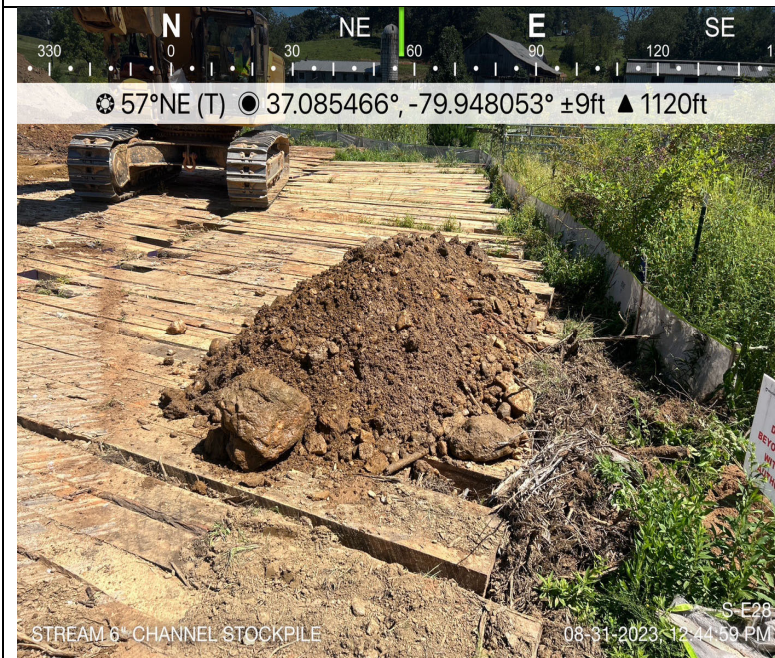
Photo Description: Channel substrate segregated and stockpiled on timber mat.
