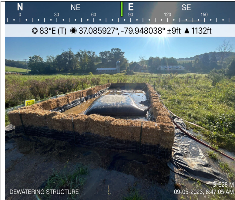
Photo Description: Dewatering structure installed and operating.
