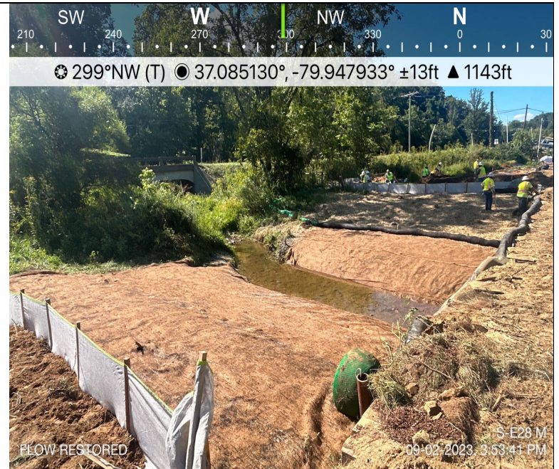
Photo Description: Restored and stabilized stream banks.
