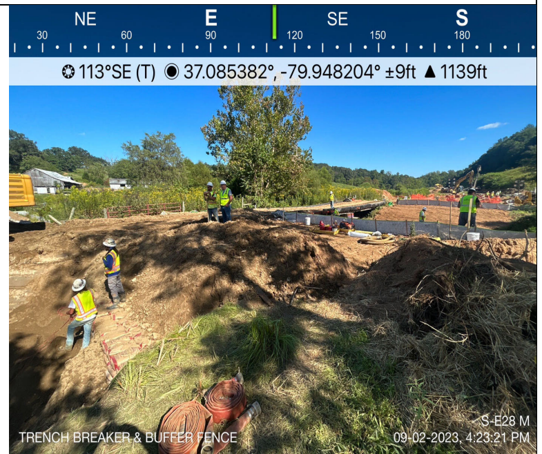
Photo Description: Trench breaker installation.
