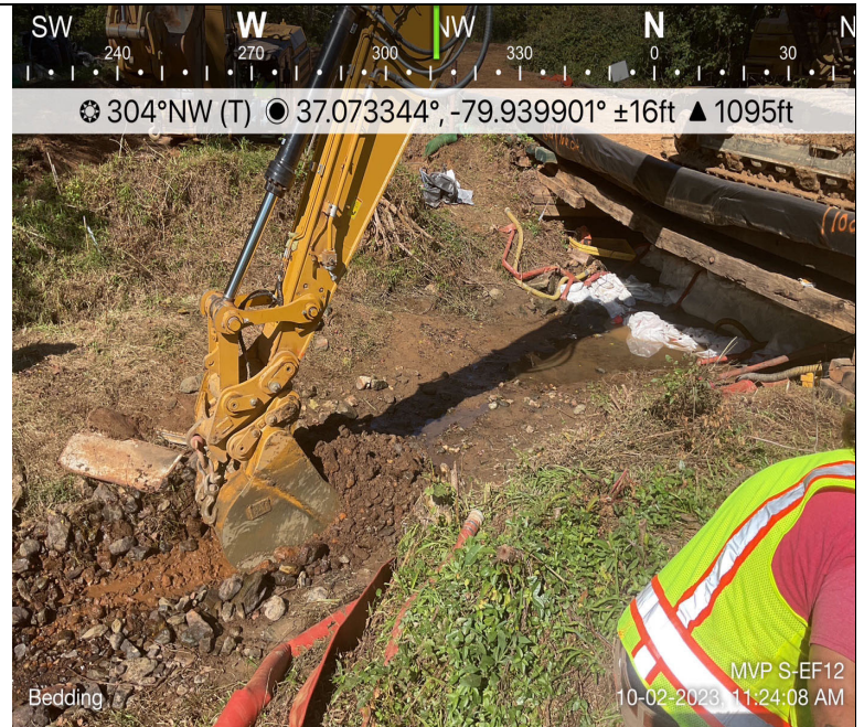
Photo Description: Streambed removal.
