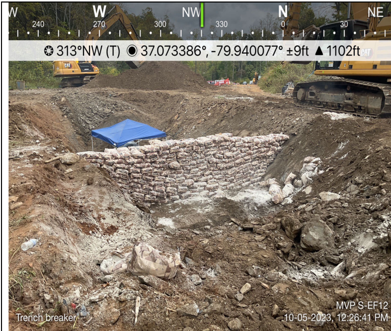
Photo Description: Trench breaker installation.
