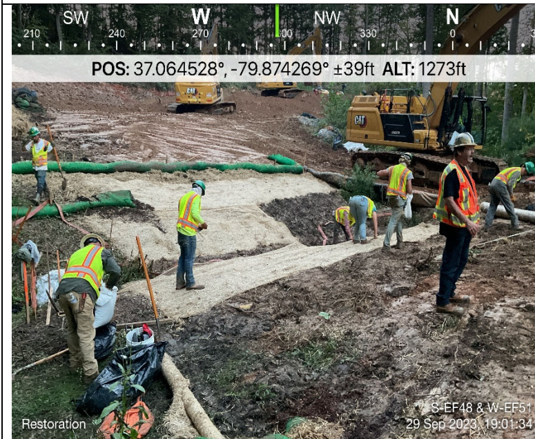
Photo Description: Restoration crews applying seed & stabilization matting to resource banks.
