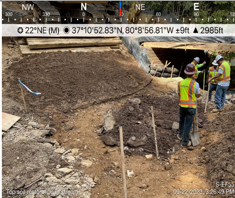
Photo Description: Restoration of topsoil and stream substrate for restoration.
