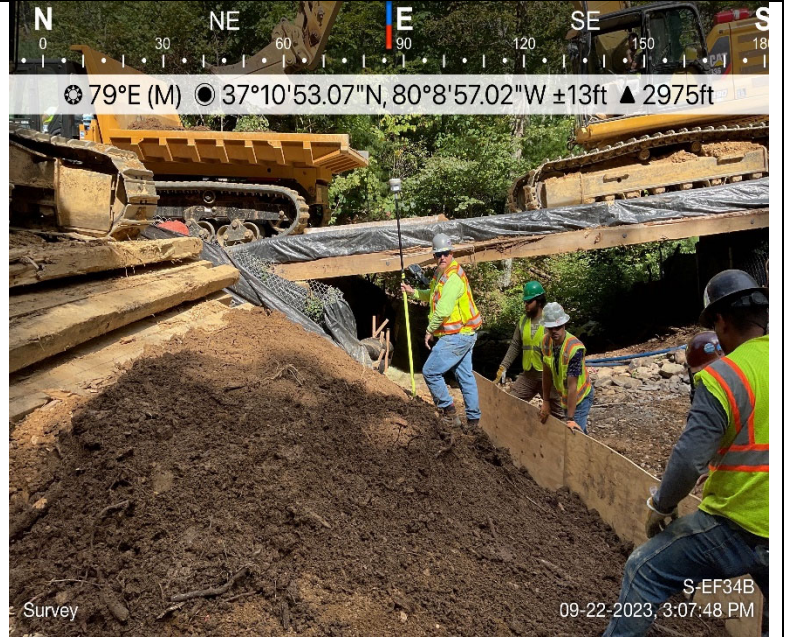
Photo Description: Survey crews staking out as-builts for restoration crews.
