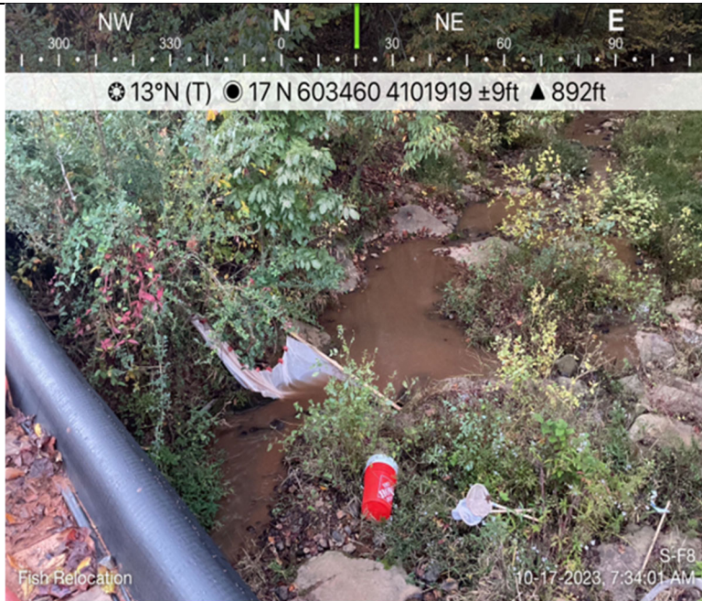
Photo Description: Downstream conditions of the resource after pump-down of upland trench to control turbidity. No fish kills or accumulated material was observed off-site.
