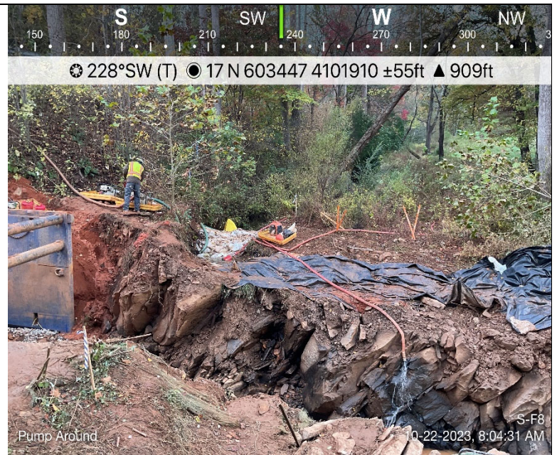
Photo Description: An overview of the pump around transporting water.
