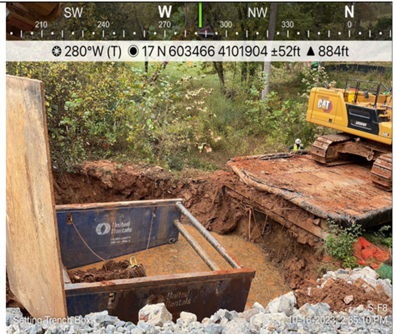
Photo Description: Upland trench excavation when turbid water emerged from bank into resource.
