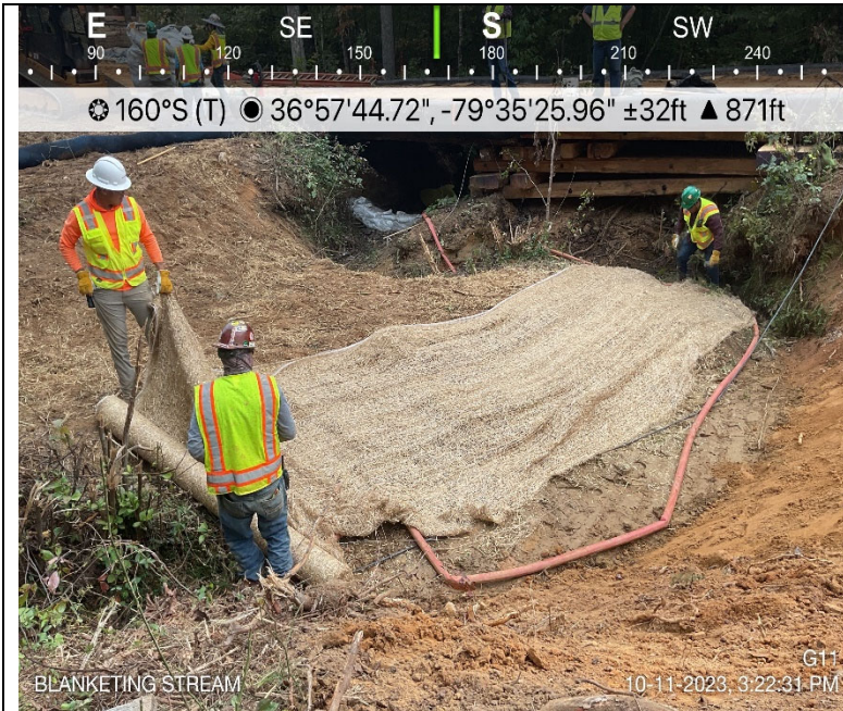
Photo Description: Erosion control matting installation during restoration.
