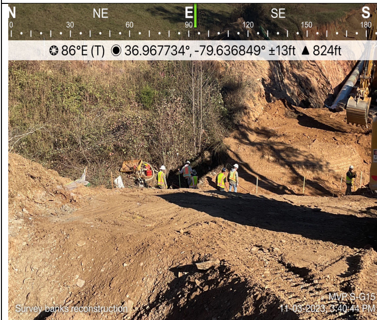
Photo Description: Survey on-site for restoration activities.
