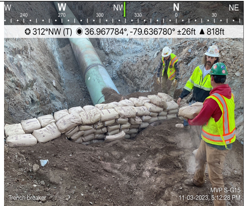
Photo Description: Trench breaker installation outside of stream banks.
