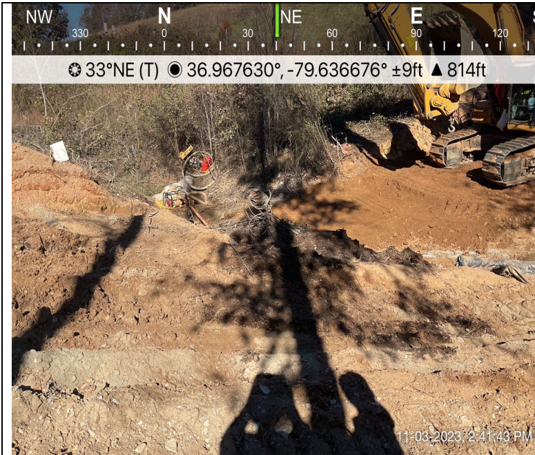
Photo Description: Dam and pump installed for duration of crossing.
