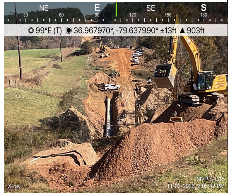
Photo Description: X-Ray QC of pipe welds.
