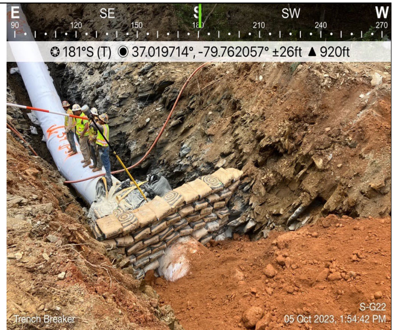
Photo Description: Trench breaker installation.
