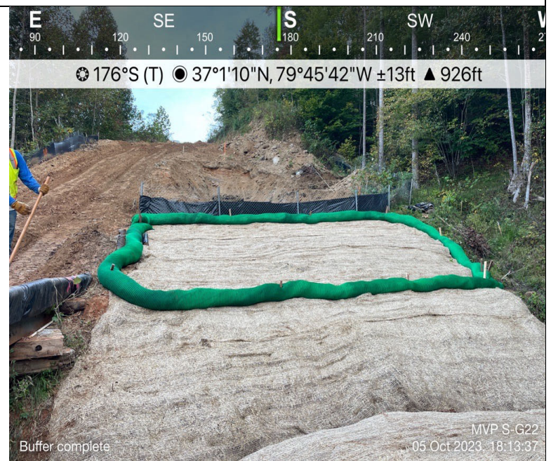
Photo Description: Completed GAS buffer zones and erosion control matting installed.
