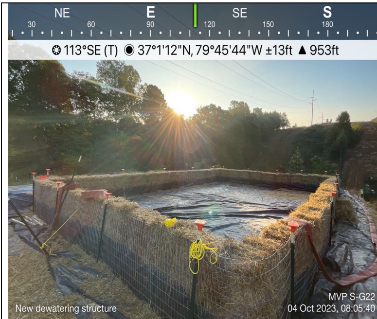
Photo Description: Dewatering structure installed for crossing.
