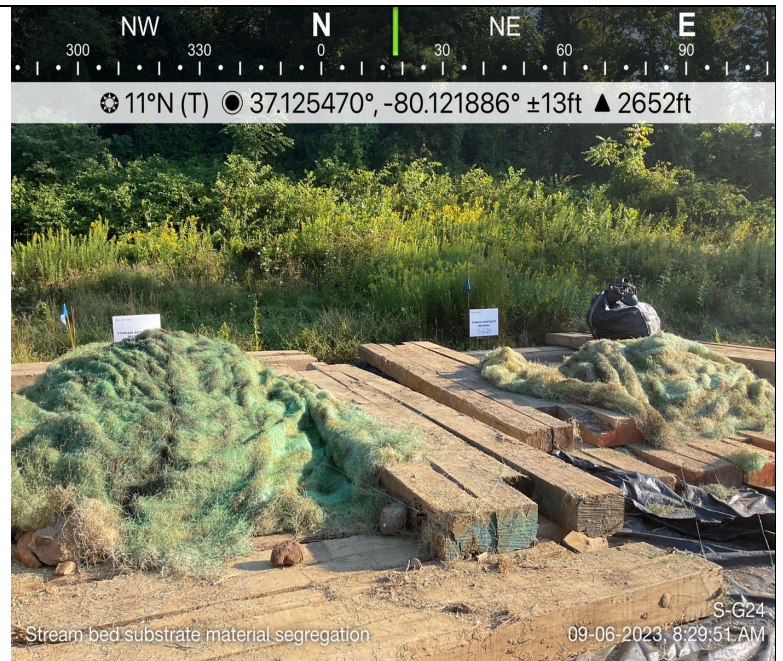
Photo Description: Streambed substrate segregated and stockpiled on timber mats.
