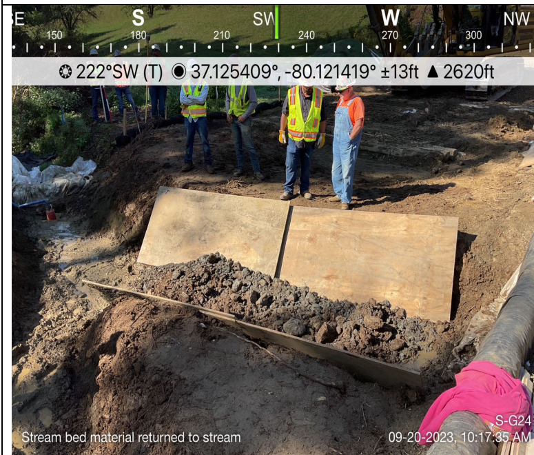
Photo Description: Rough backfill and grading of stream channels.
