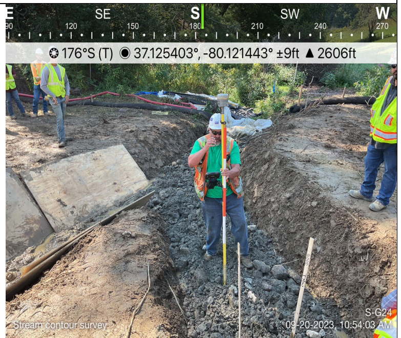
Photo Description: Survey crew on-site assisting with stream contours during restoration.
