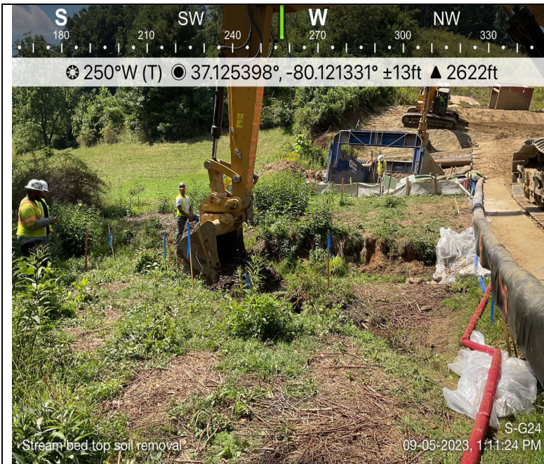
Photo Description: Stripping of topsoil and stream substrate for stockpiling.
