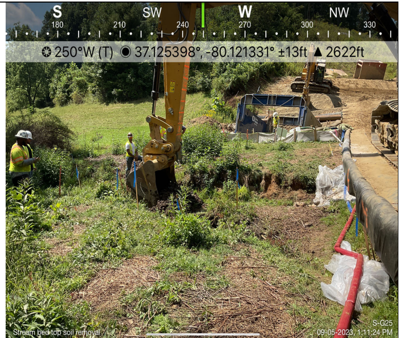
Photo Description: Topsoil removal within resource impact area.
