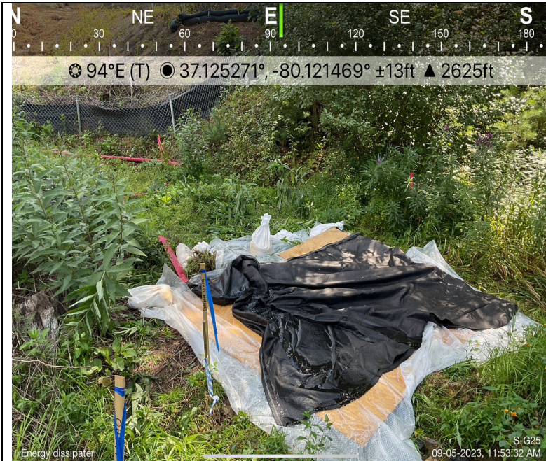
Photo Description: Dam and pump around energy dissipator installed and functioning.
