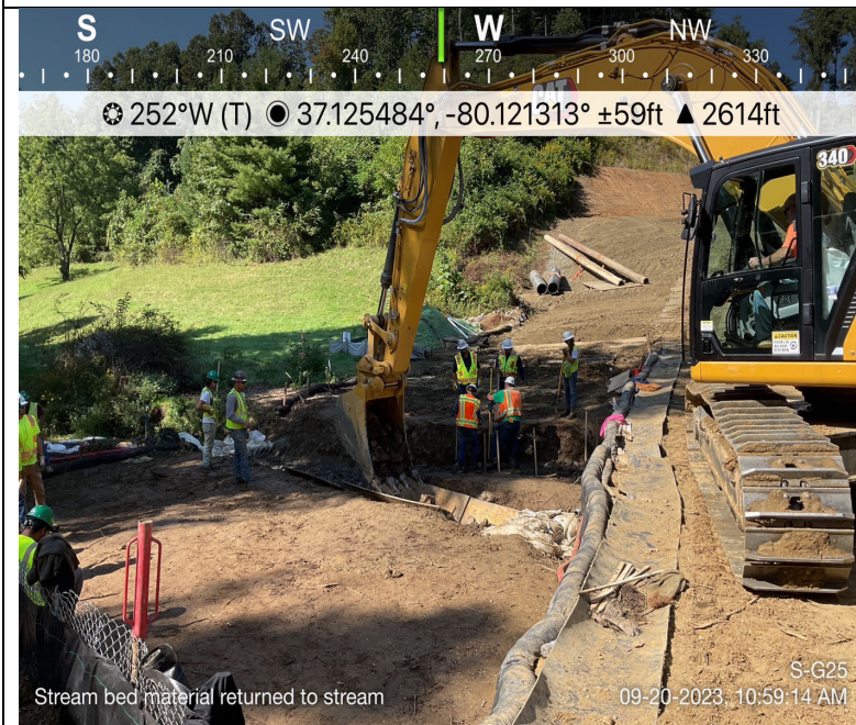
Photo Description: Restoration of streambed material into the resource.
