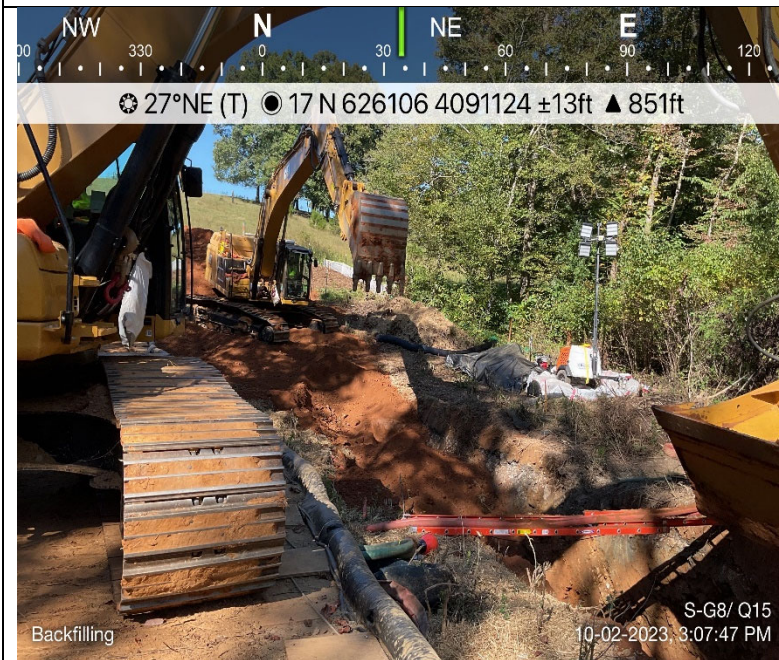
Photo Description: Backfilling of subsoil to resource area.
