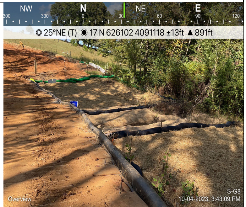
Photo Description: Overview of restored resource area post-construction.
