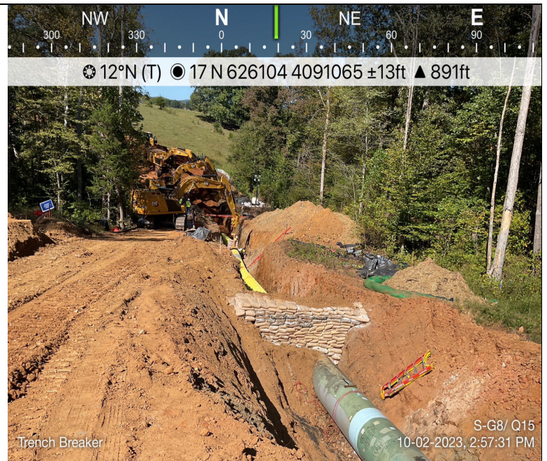
Photo Description: Trench breakers installed.
