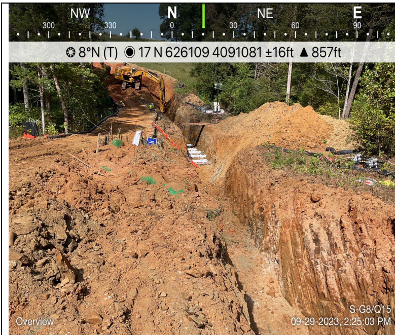
Photo Description: Installing padding for pipe.
