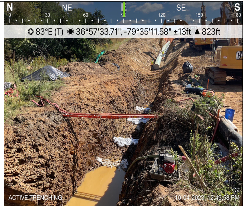
Photo Description: Dam and pump operational throughout crossing.
