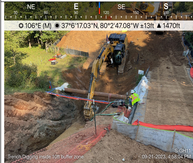
Photo Description: Trench excavation through resource.
