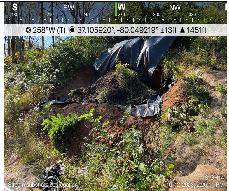
Photo Description: Stream substrate segregation.
