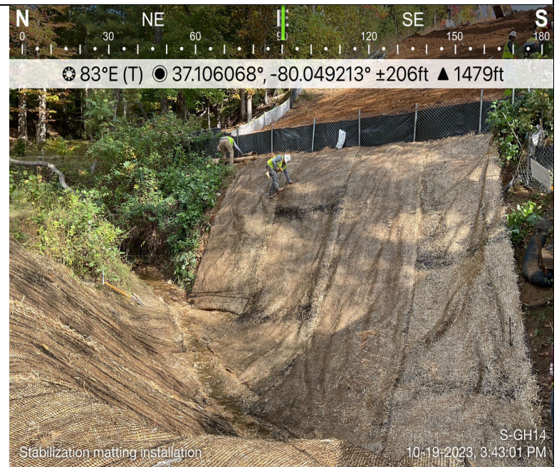
Photo Description: Heavy duty stabilization matting and high velocity screw pins.
