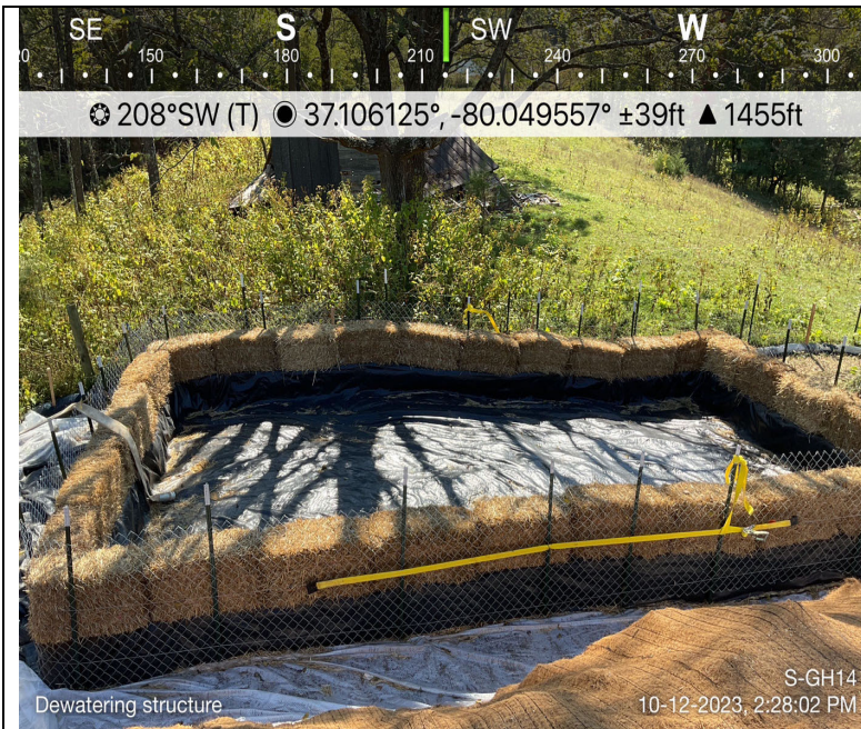
Photo Description: Dewatering structure.
