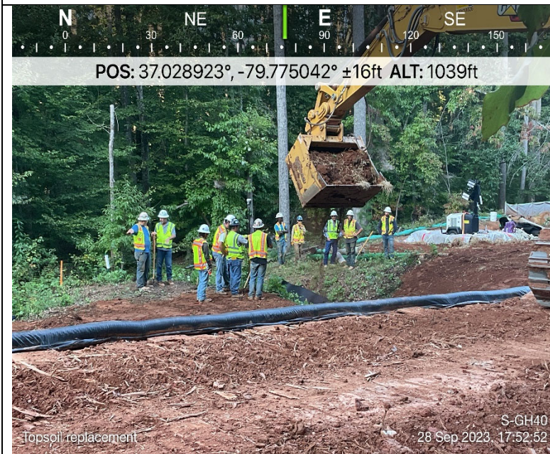
Photo Description: Topsoil restoration.
