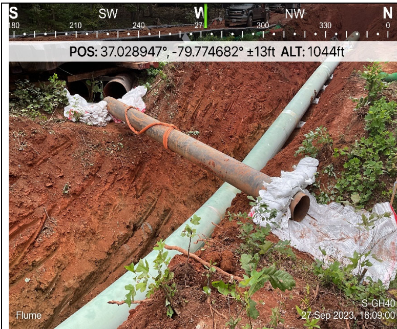
Photo Description: Flume crossing installed and functioning throughout crossing.
