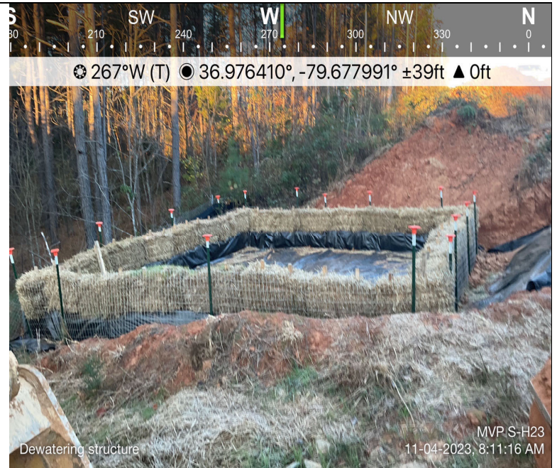
Photo Description: An overview of the dewatering structure.
