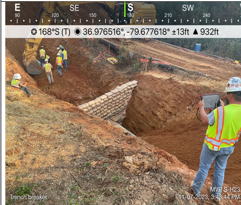
Photo Description: A trench breaker installed for the resource.
