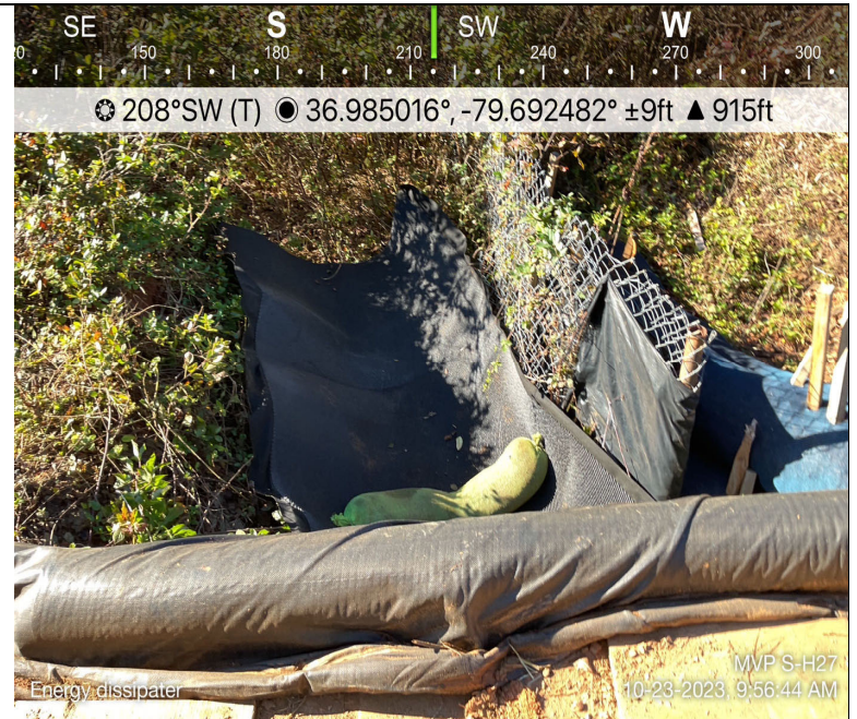
Photo Description: Energy dissipater installed on site.
