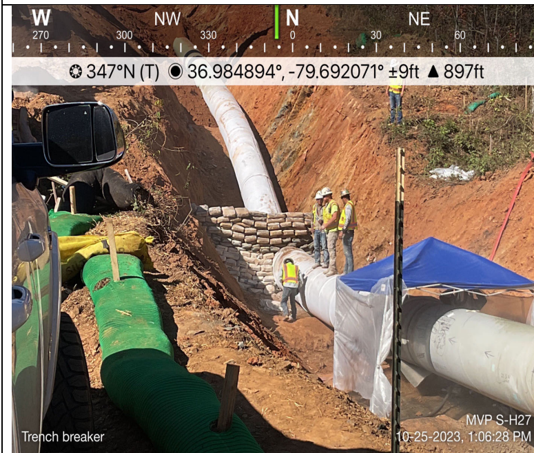
Photo Description: Installation of a trench breaker.
