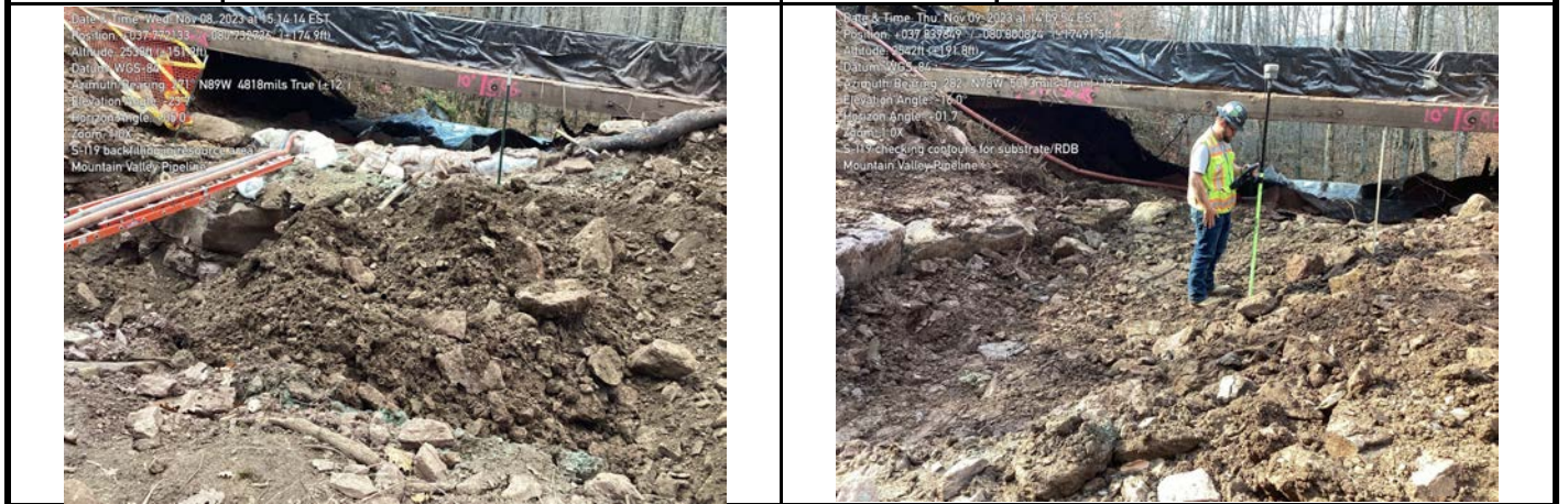
GPS Location See Photo GPS Location See Photo Description Photo 7: Backfilling in aquatic resource area. Description Photo 8: Survey marking contour elevations.
