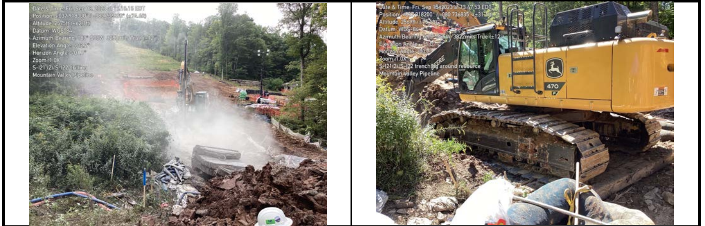
GPS Location See photo GPS Location See photo Description Photo 3: Drilling in aquatic resource area. Description Photo 4: Trenching in aquatic resources.
