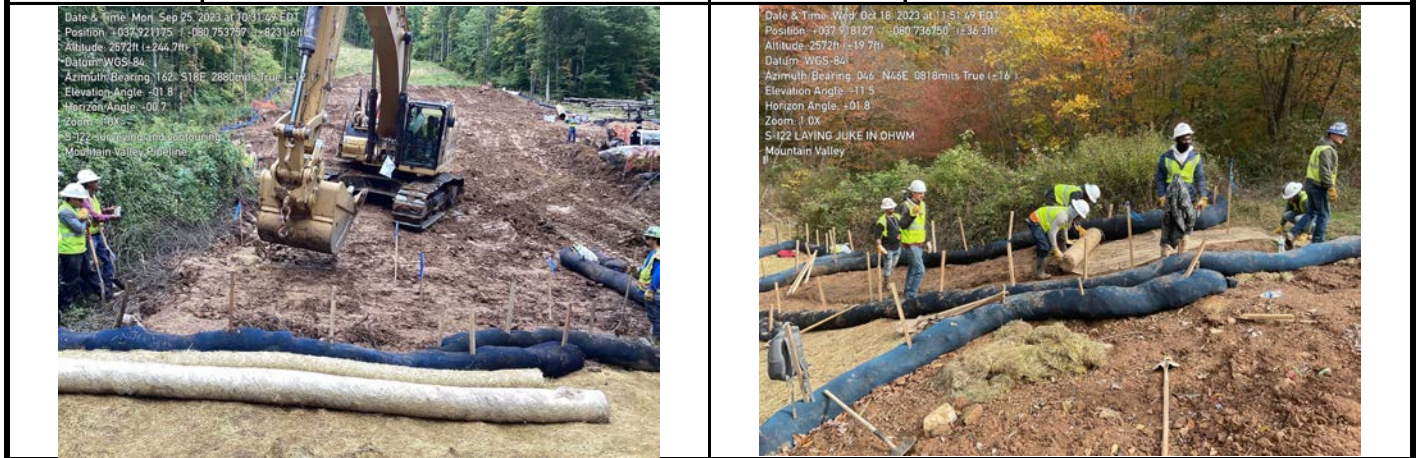
GPS Location See photo GPS Location See photo Description Photo 7: Survey being completed and contours being restored. Description Photo 8: Spreading jute matting after stream is reworked by hand.
