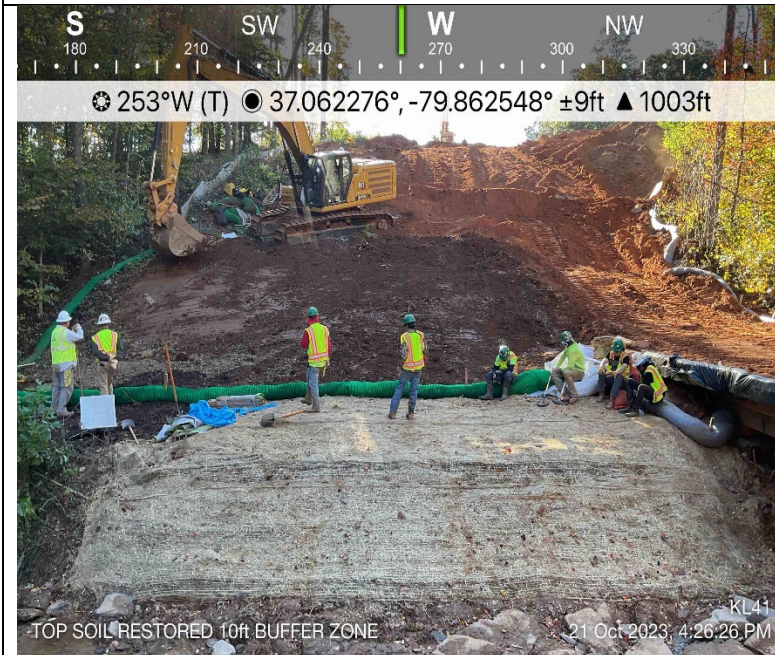
Photo Description: Restoration of the topsoil adjacent to the stream. Seed and stabilization matting installed along streambanks.
