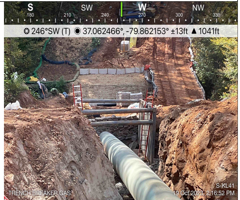
Photo Description: Trench breaker in GAS.
