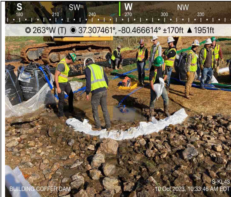
Photo Description: Cofferd dam inside of dammed area.
