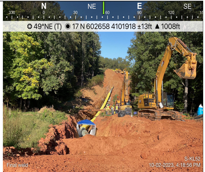
Photo Description: Trench excavated, and pipe lowered in.
