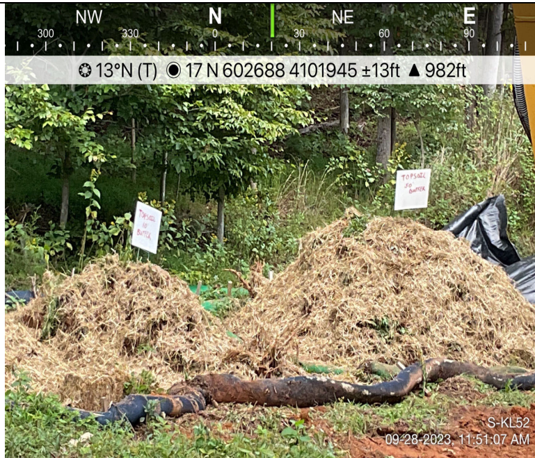
Photo Description: Topsoil stockpiles with stabilization.
