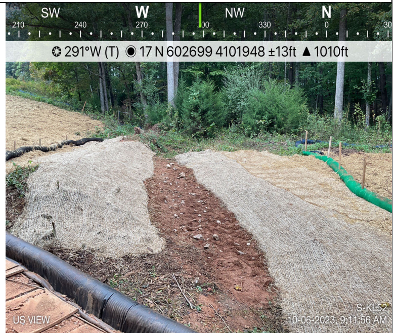
Photo Description: Restoration and stabilization of resource impact area.
