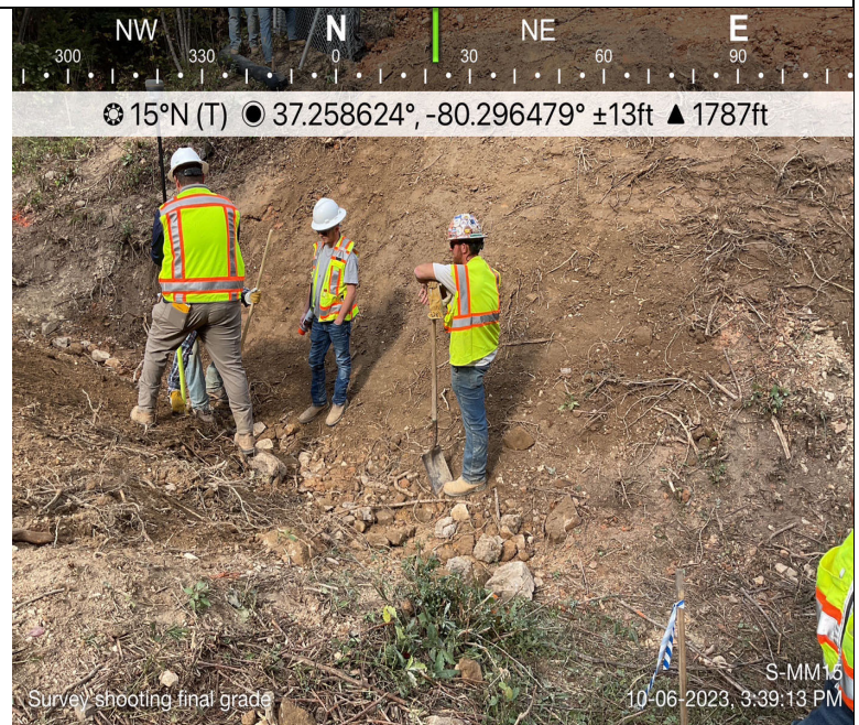
Photo Description: Final grade survey shots.
