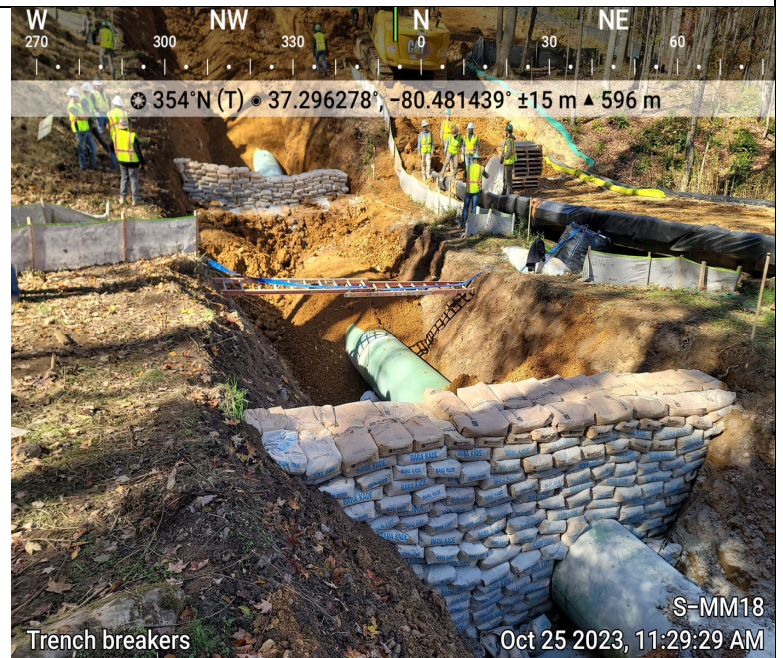
Photo Description: Trench breakers installed over the pipe.
