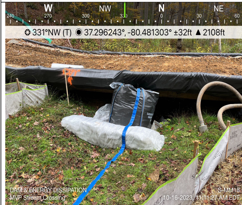
Photo Description: Dam and energy dissipation bag.
