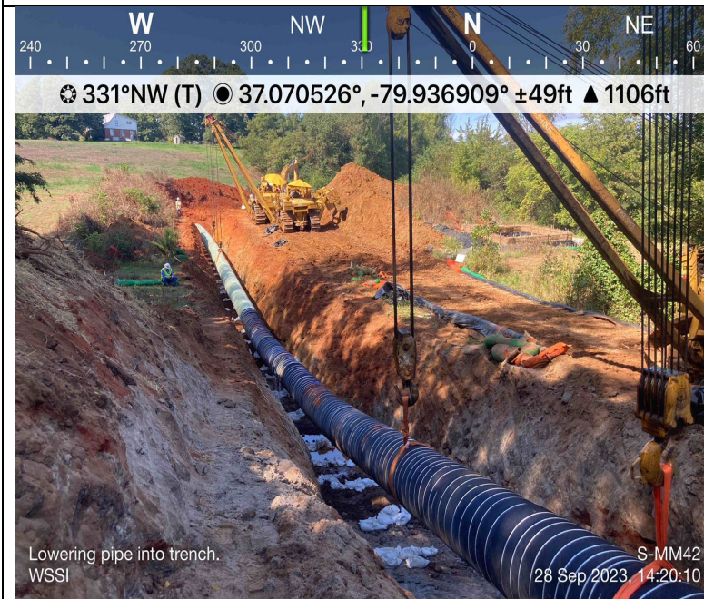
Photo Description: Pipe lowering in to resource.
