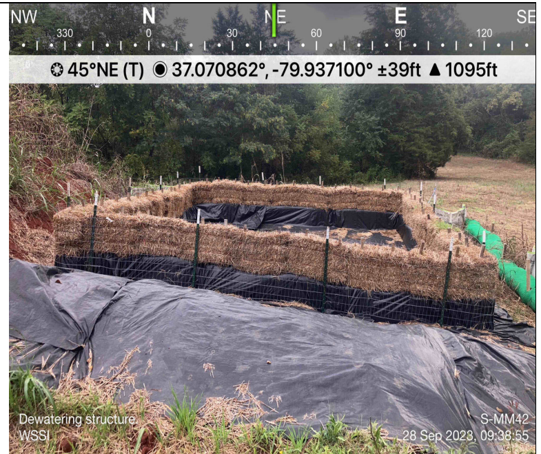
Photo Description: Dewatering structure
