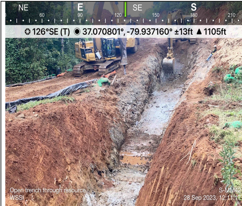
Photo Description: Open trench through resource.
