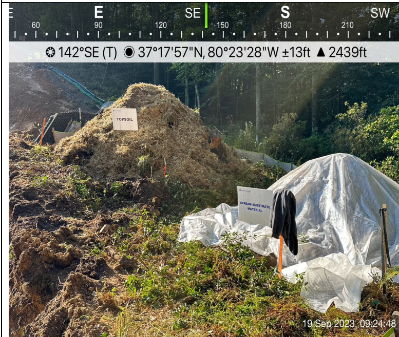
Photo Description: Soil and streambed stockpiles.
