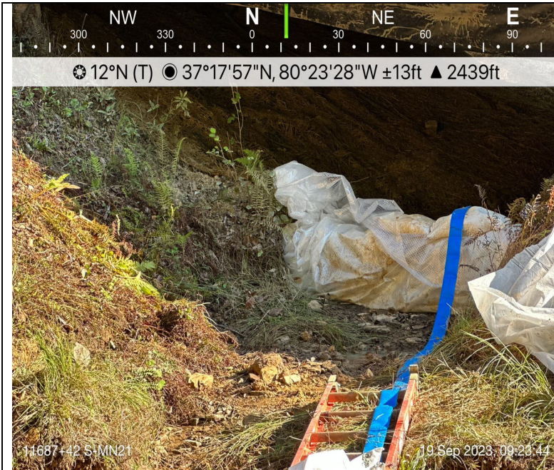
Photo Description: Dam & pump installed and operated throughout crossing.
