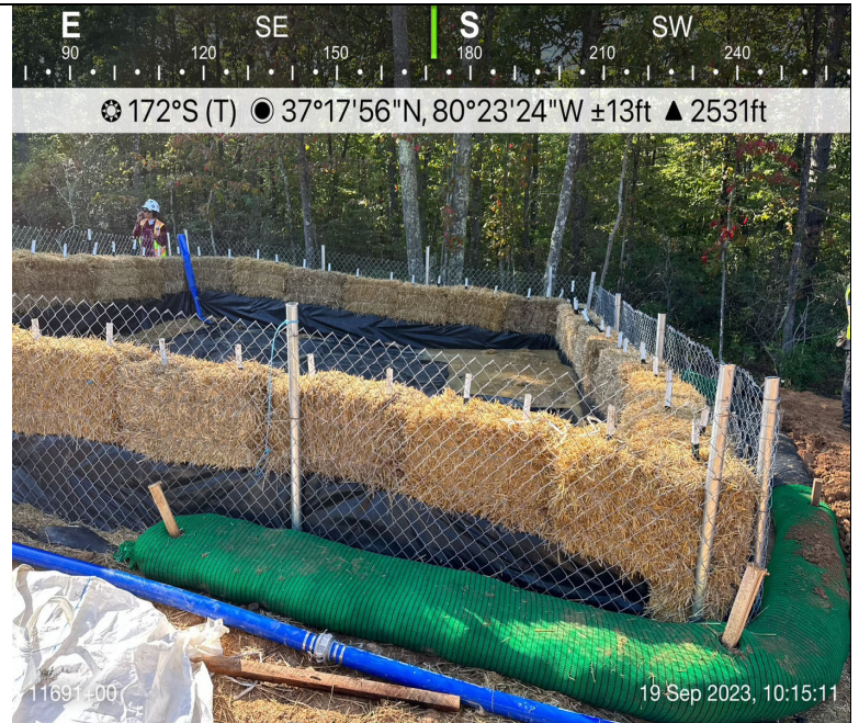
Photo Description: De-watering structure set up for use throughout crossing.
