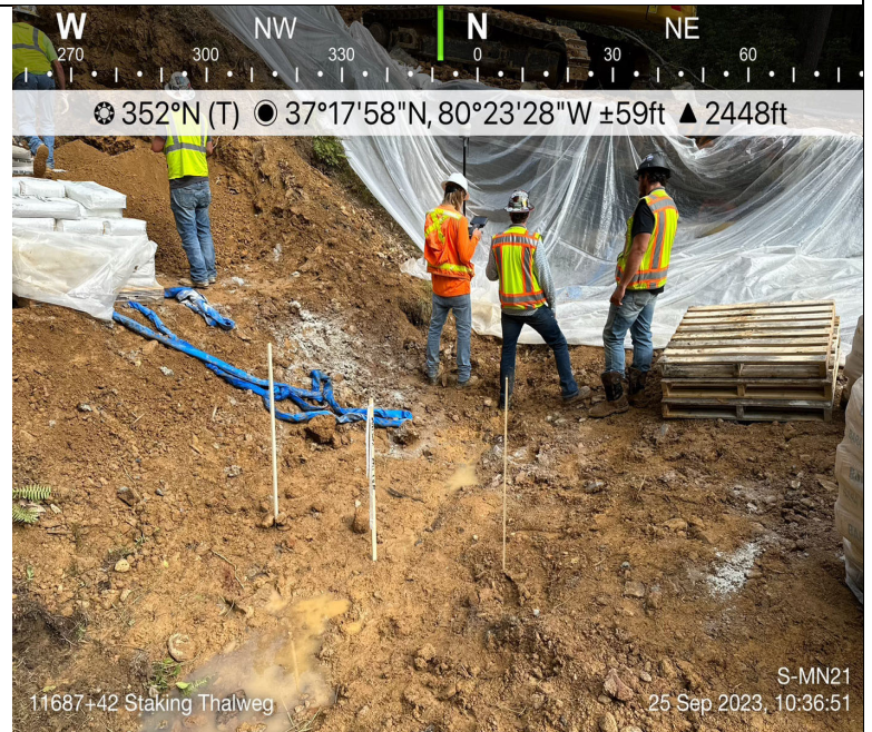
Photo Description: Survey stake out for restoration crews.
