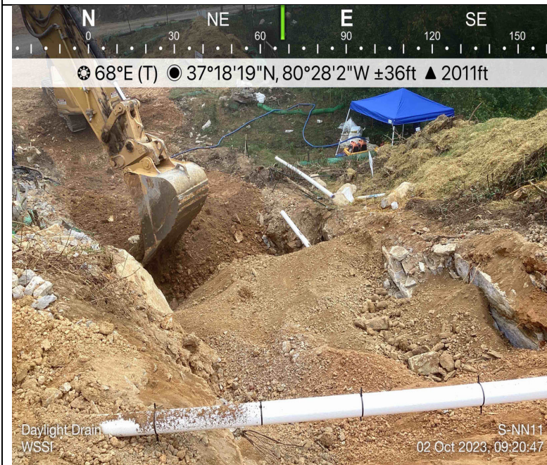
Photo Description: Daylight drain installed.
