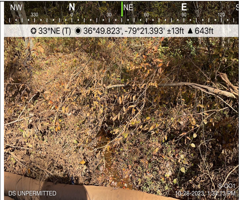
Photo Description: Conditions of the downstream area outside the ROW during pre-construction assessment.
