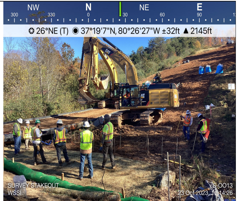
Photo Description: Survey staking out final contours.
