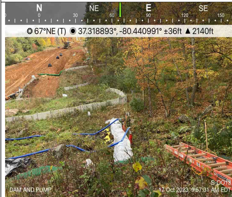
Photo Description: Dam and pump around installed.
