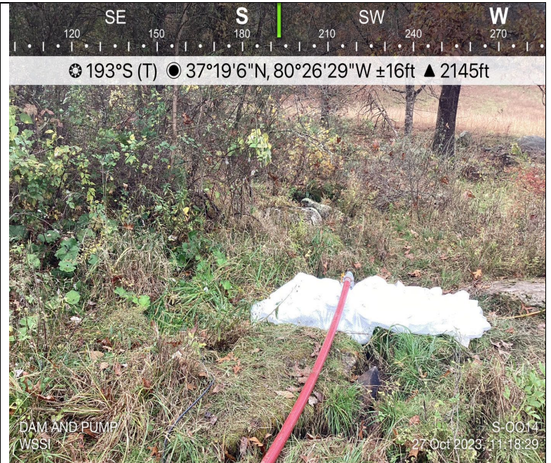
Photo Description: Dam and pump installed and functioning.
