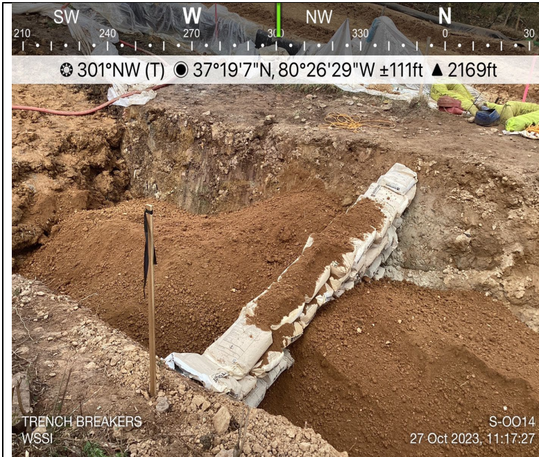
Photo Description: Trench breakers installed.
