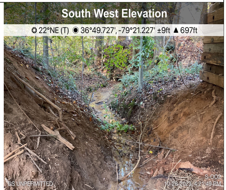
Photo Description: Conditions of the downstream area outside the ROW during post-construction assessment.
