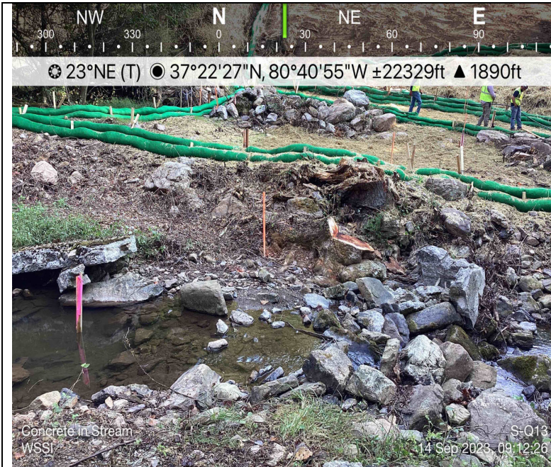
Photo Description: Pre-existing concrete to be removed and disposed of properly.
