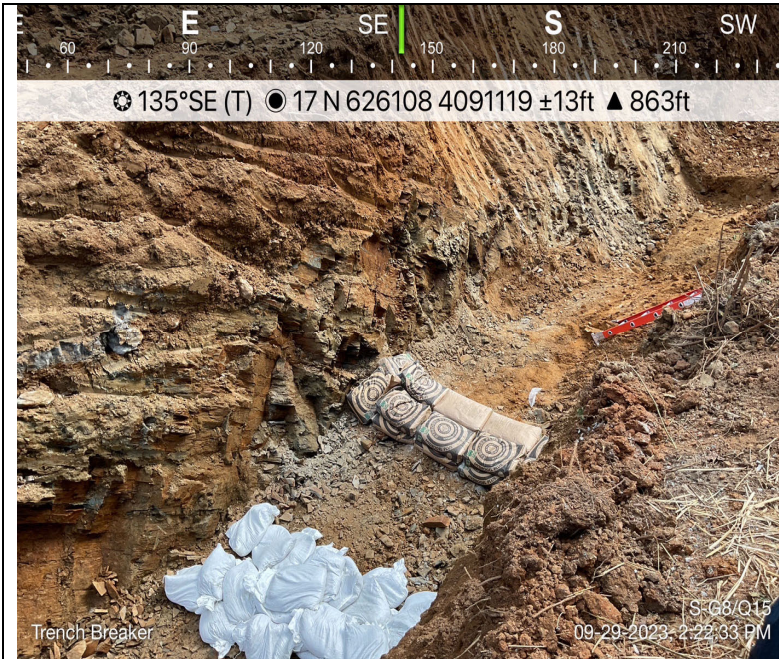
Photo Description: Installation preparation for trenchbreakers.
