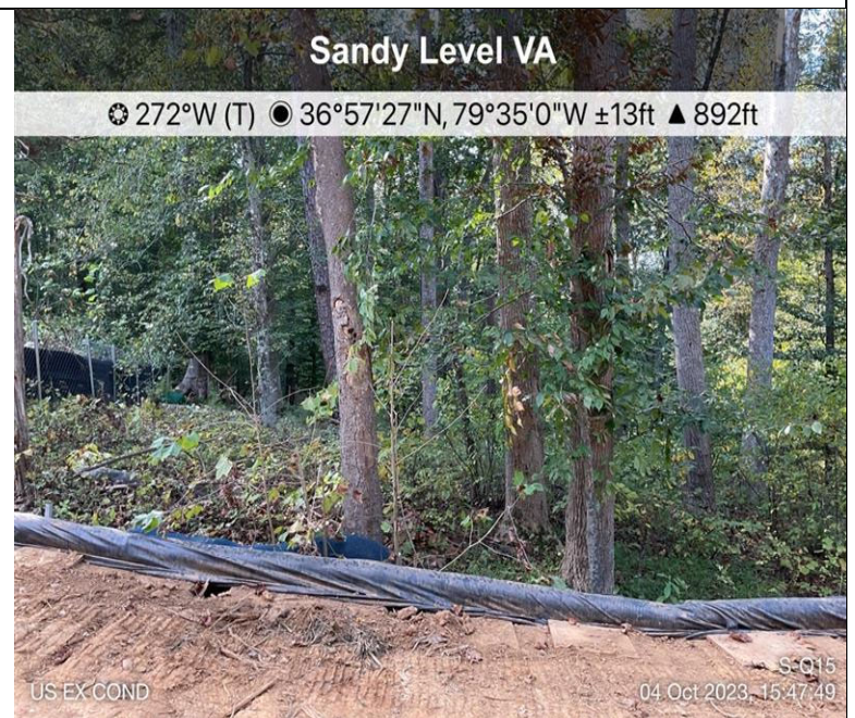
Photo Description: Conditions of the downstream area outside the ROW during post-construction assessment. Typo in photo watermark — “DS* EX COND”
