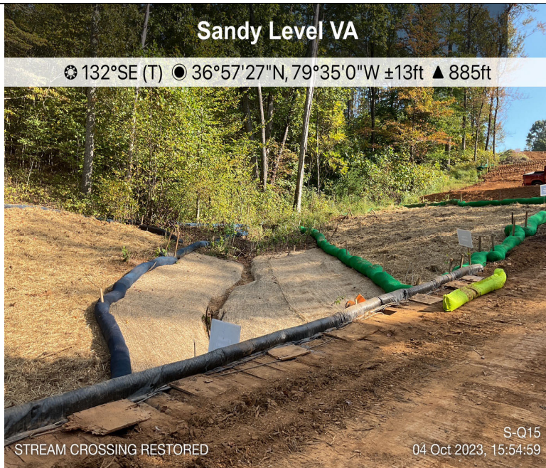
Photo Description: Stream crossing completed and restoration complete.
