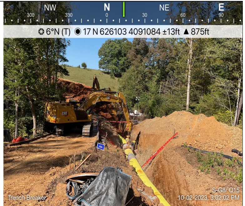
Photo Description: Pipe lowered into trench.
