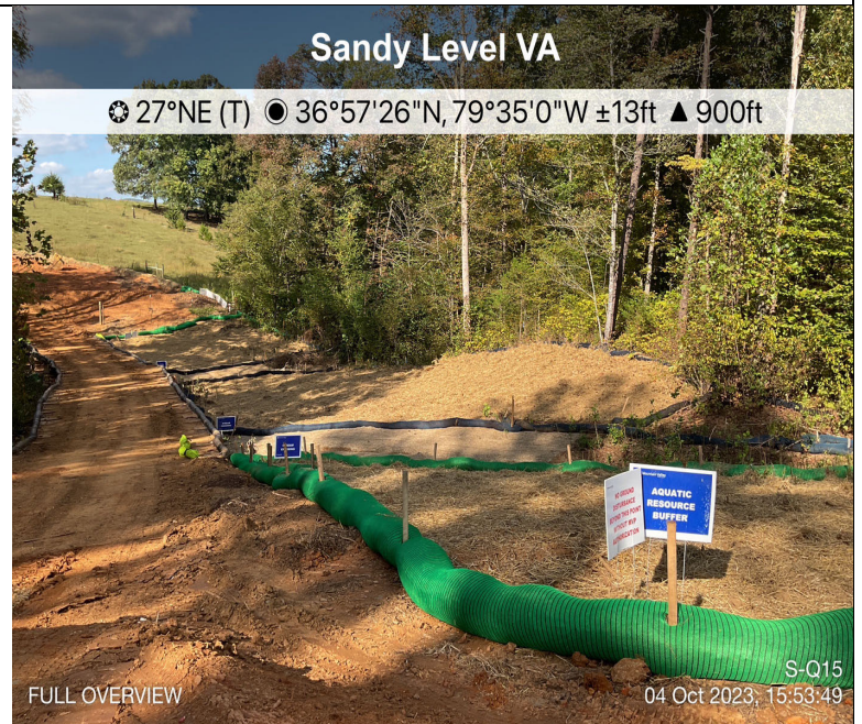
Photo Description: Travel lane remains installed/active. Resource area restoration/revegetation overview.
