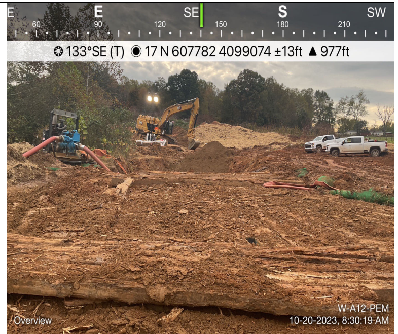
Photo Description: Timber mats used during the resource crossing.
