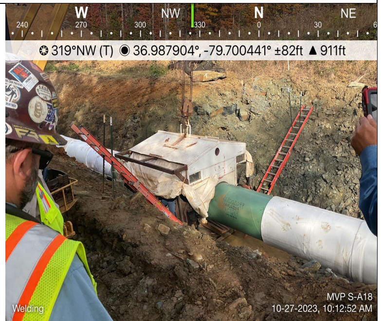
Photo Description: Welding pipe within trench.
