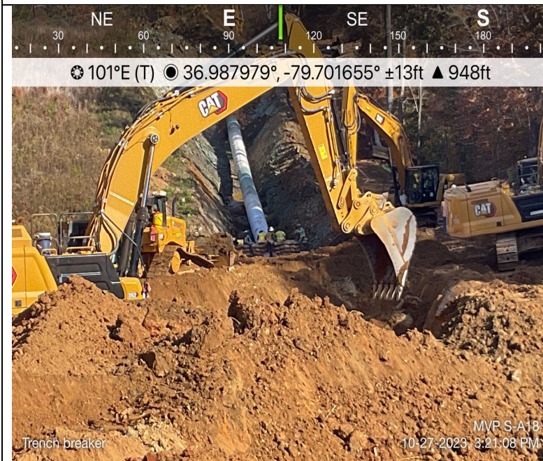
Photo Description: Trench breaker installation.
