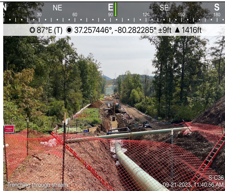
Photo Description: Trenching through resources.
