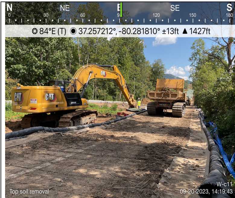
Photo Description: Top soil removal in wetland.
