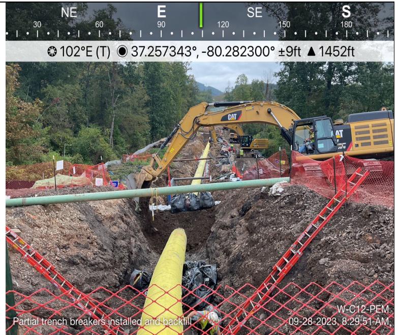
Photo Description: Trench breakers within 25 of the resources.
