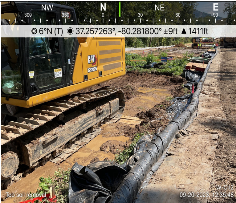
Photo Description: Wetland top soil removal.
