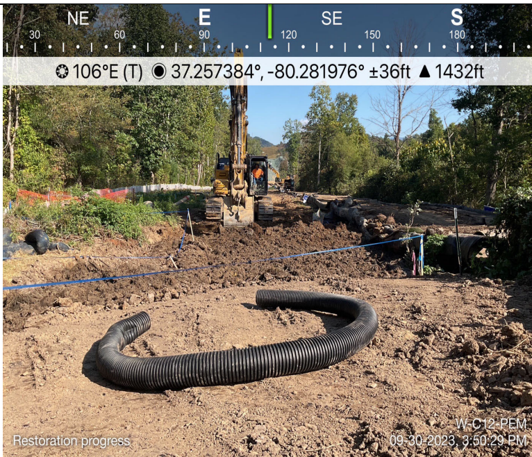
Photo Description: Top soil restoration of wetland.
