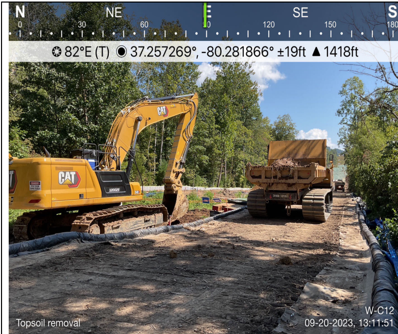
Photo Description: Top soil removal through wetland.
