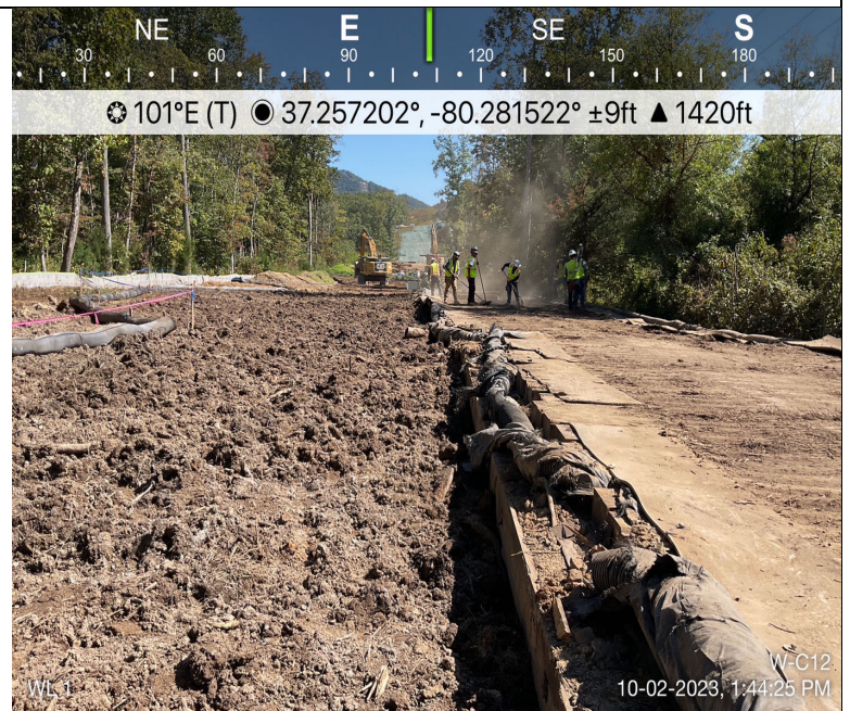
Photo Description: Final restoration and seeding of wetlands.
