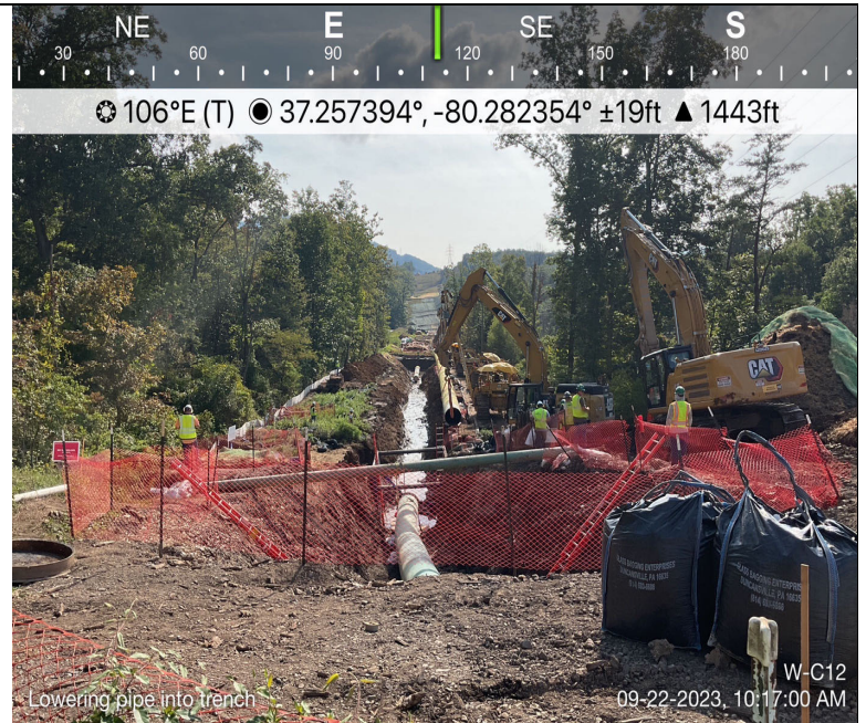
Photo Description: Pipe installation into trench.
