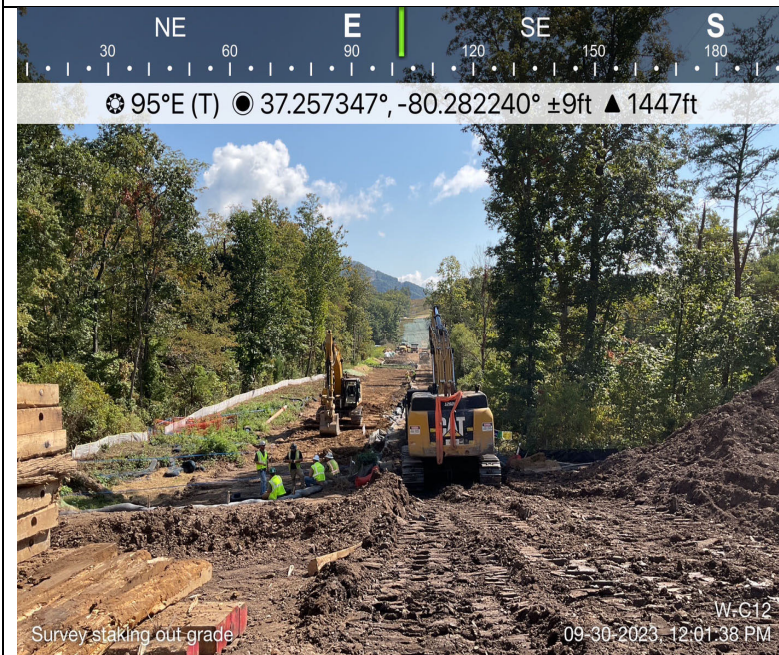
Photo Description: Survey staking out for final grade and wetland boundaries.
