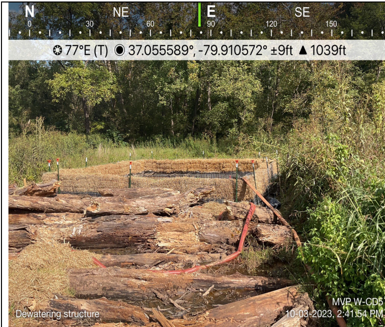
Photo Description: Dewatering structure for trenching
