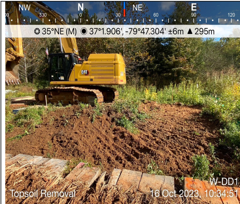
Photo Description: Removing top 12 inches of topsoil from W-DD1.
