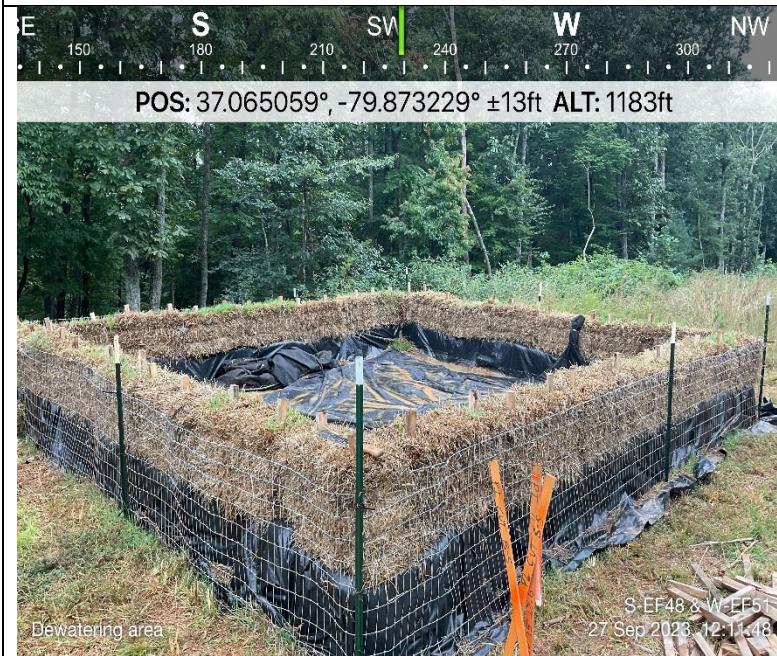
Photo Description: Dewatering operation/structure installed and operational during crossing.
