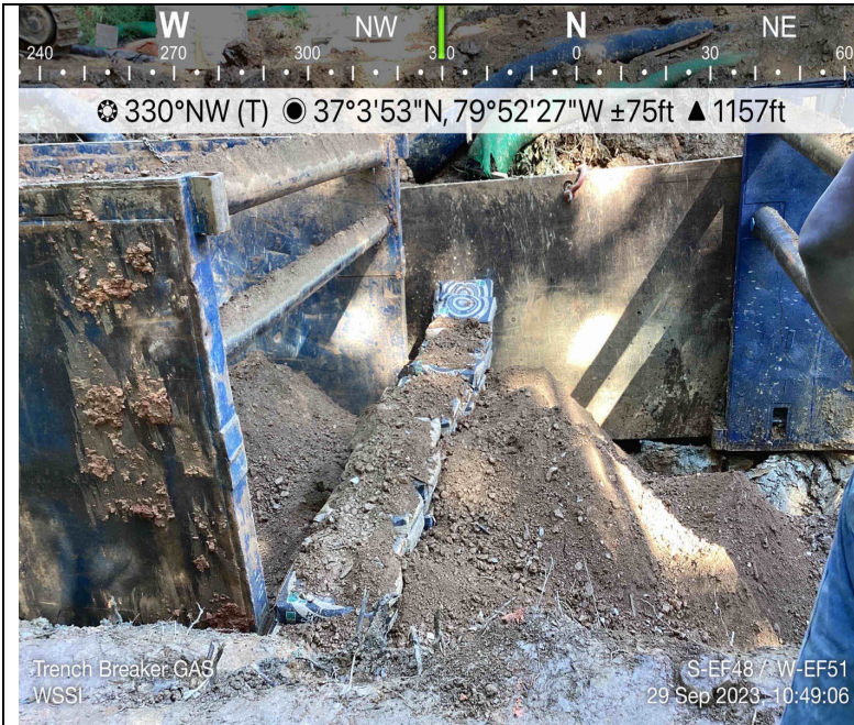
Photo Description: Trenchbreaker installed on going away side of resource.
