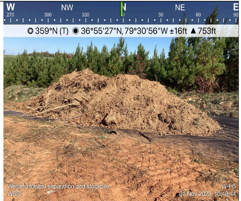
Photo Description: Wetland topsoil that has been separated and stockpiled.
