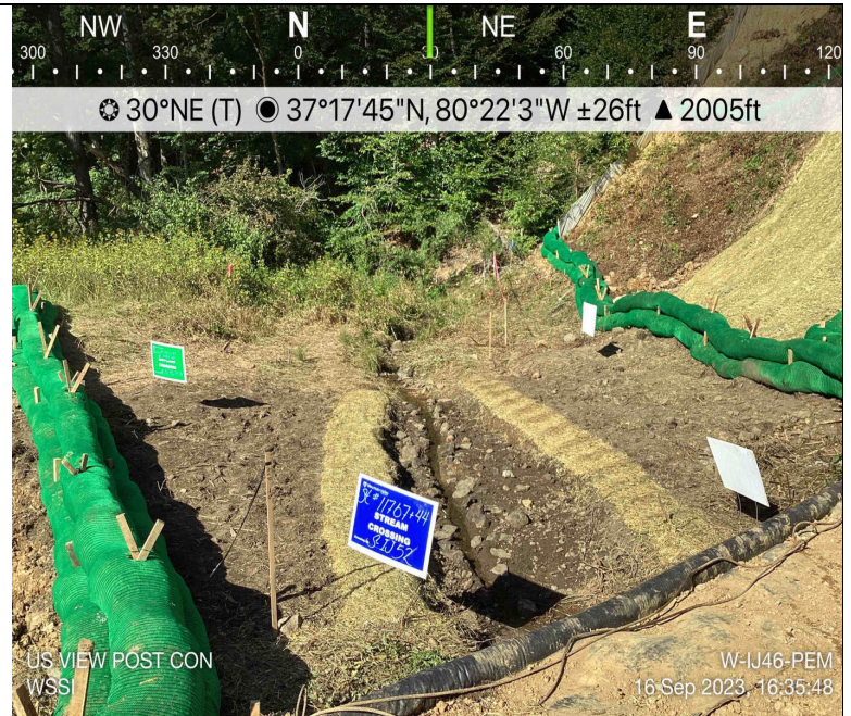
Photo Description: Upstream view of stream and wetland crossing post construction.
