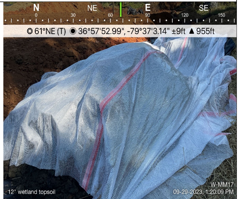
Photo Description: Wetland topsoil stockpiled and wrapped separately from subsoils.
