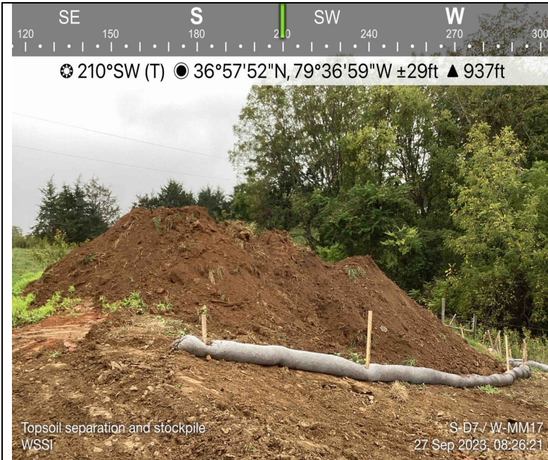
Photo Description: Buffer zone topsoil stockpiled separately from wetland topsoil.
