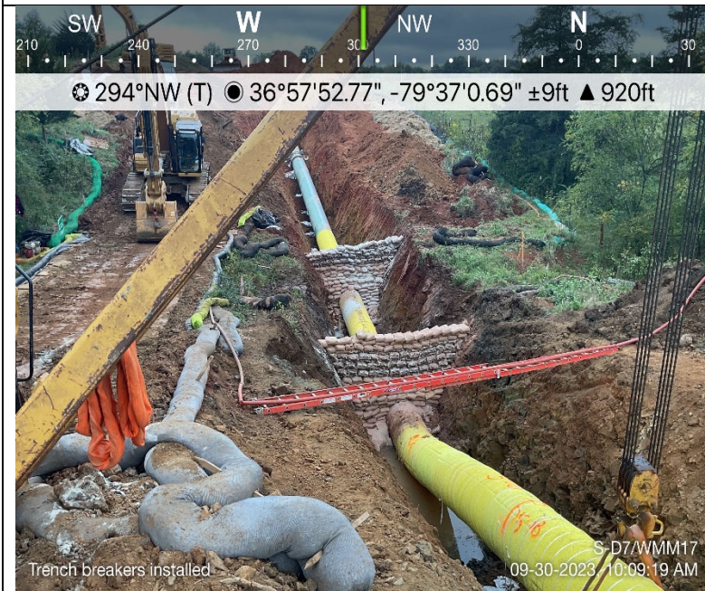
Photo Description: Trenchbreaker installations.
