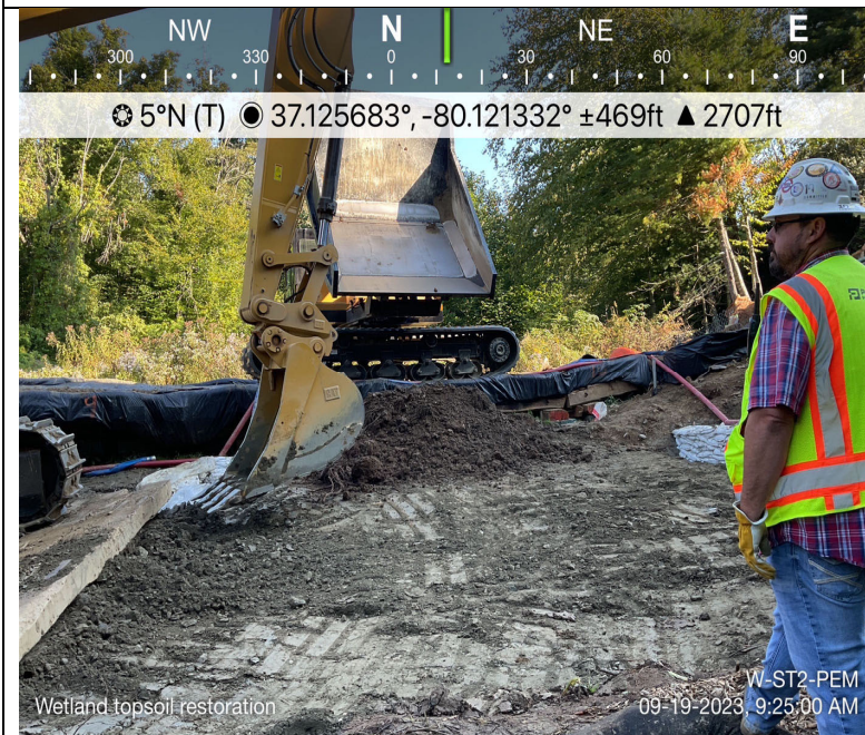
Photo Description: Restoring wetland topsoil.
