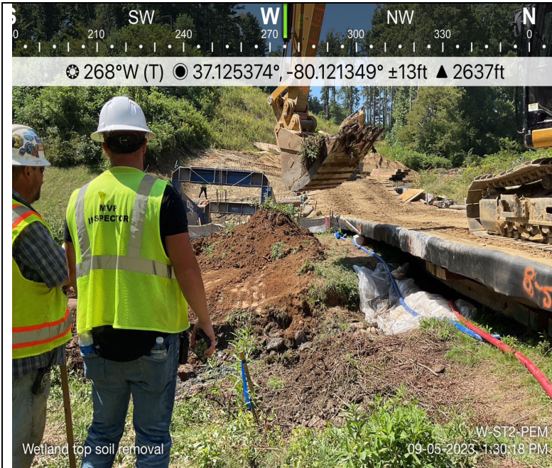
Photo Description: Wetland topsoil removal prior to trenching.
