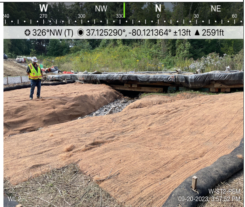
Photo Description: View of final stabilization and restoration of work area.
