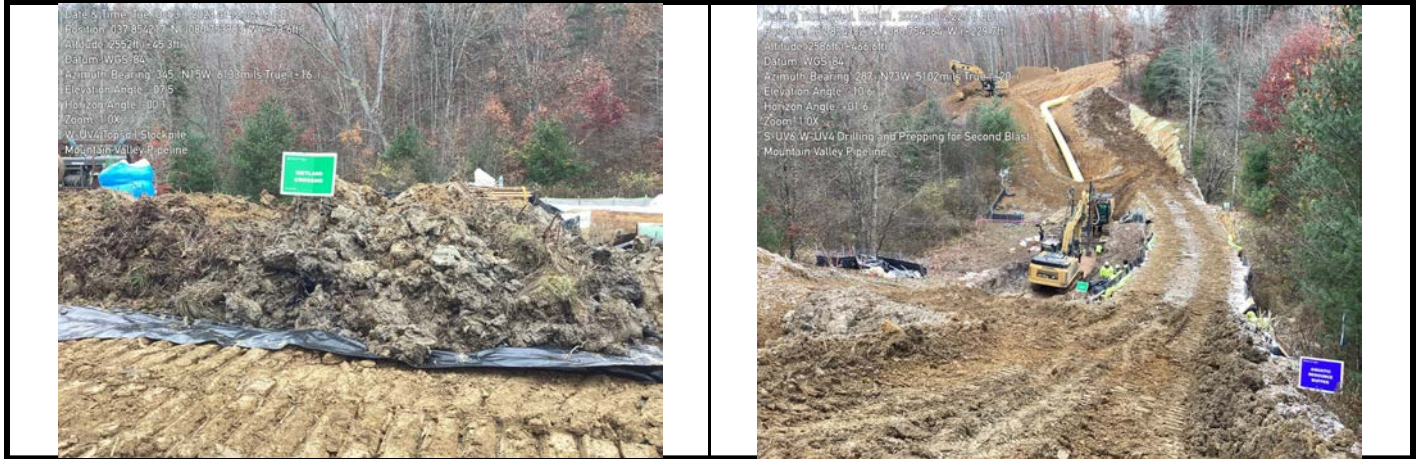
GPS Location See Photo GPS Location See Photo Description Photo 3: Wetland topsoil segregated in upland area. Description Photo 4: Prepping (drilling) for second blast.
