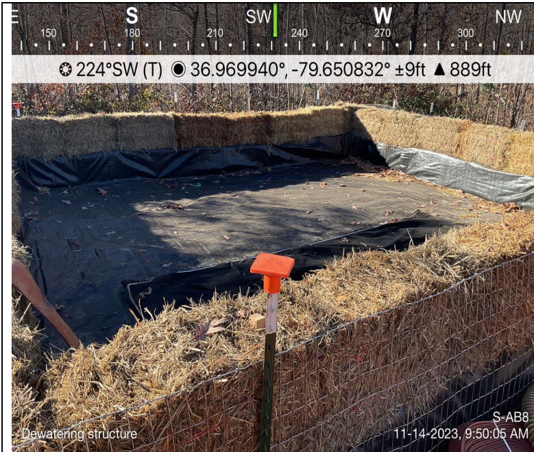
Photo Description: Dewatering structure
