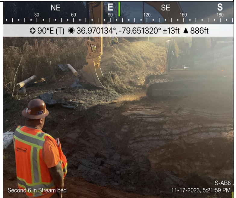
Photo Description: Second 6 inch of stream bed material
