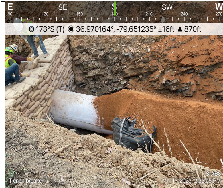
Photo Description: Trench breaker
