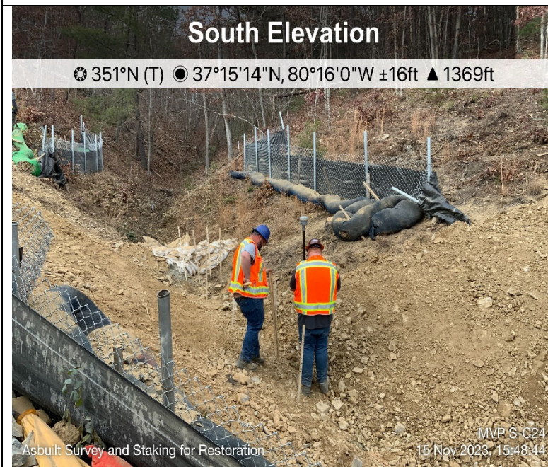
Photo Description: Survey staking out for restoration.
