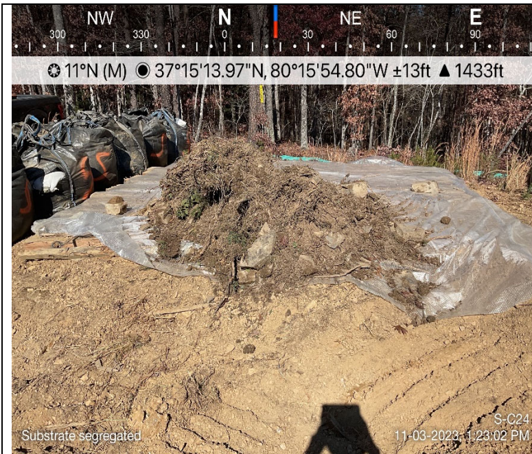
Photo Description: Streambed substrate/topsoil was stripped and segregated.
