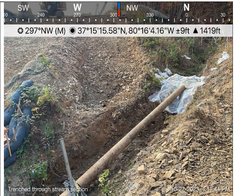
Photo Description: Flume pipe installed and operational throughout crossing.
