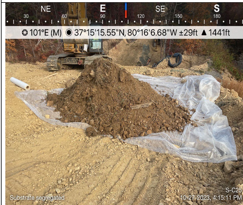
Photo Description: Streambed substrate stockpiled separately from subsoil.
