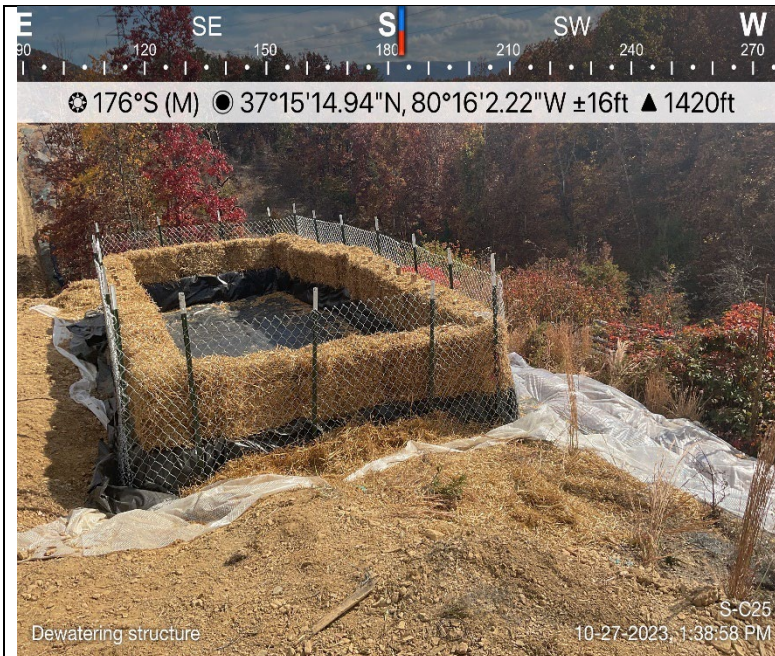
Photo Description: Dewatering structure installed and functional throughout crossing.
